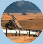
Leakage monitoring of valves and pipelines
