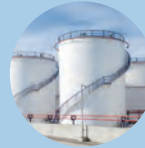
Corrosion detection of storage tanks
